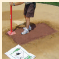
Apply a thin layer of Professional Mound Clay (match color to blocks) moisten, tamp.
