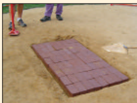
Install MOUNDMASTER Blocks, tamp, water and allow to soak in for 20 minutes.
