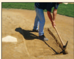
Excavate the Batter's Box 3" deep.
