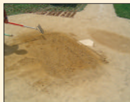
Cover with a thin layer of infield mix to finish grade.
